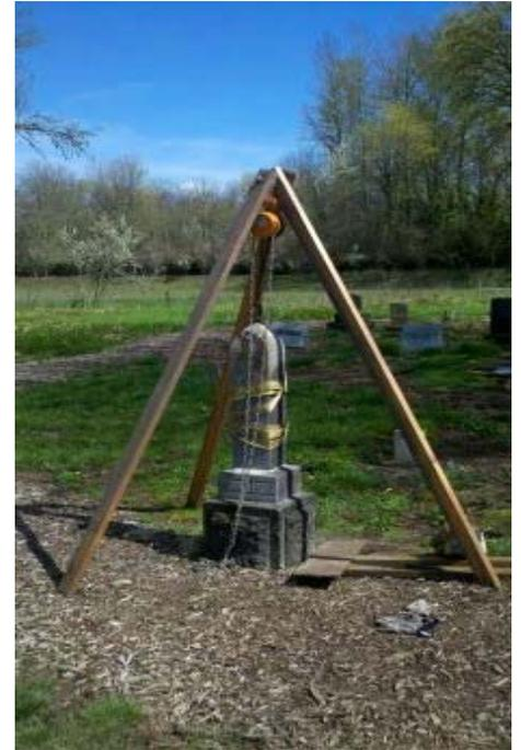
**The above Edwards marker** was vandalized in May – tipped off onto the ground. Minor damage resulted. The repair work involved lifting it back onto its base with a tripod and affixing it with epoxy. This vandalizing was most likely a late night event. The Luper board asks that everyone in the Luper network spread the word about the importance of protecting the cemetery.
